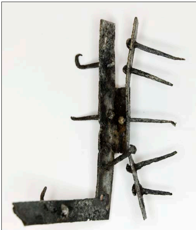
Figure 103: Hardware from the parsonage door: H-L hinge, with clinched nails; oval door pull and stem of brass
