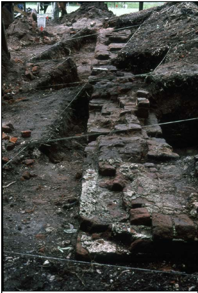
Figure 57: Southern wall of structure, facing west
