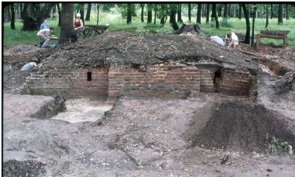
Figure 59: Completed excavations, 2005, facing the west side of the structure; note displacement of SW corner due to cracking along vent opening.
