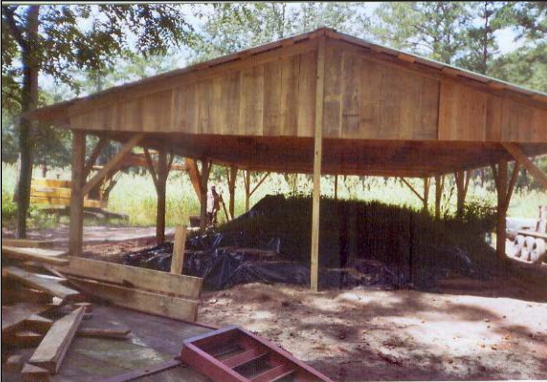
Figure 73: protective shed over the parsonage foundation, after completed excavations
